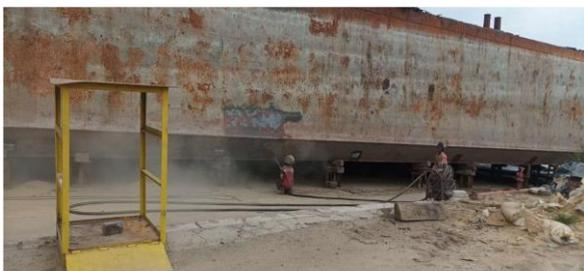
Gambar 5. Proses *Sandblasting*
