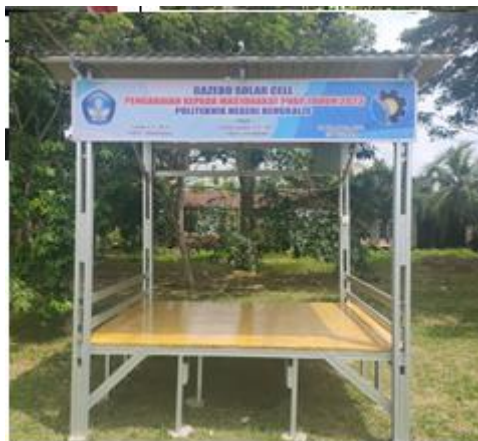
Gambar 9. Bangunan Gazebo Solar Cell (Adam, dkk, 2023)
