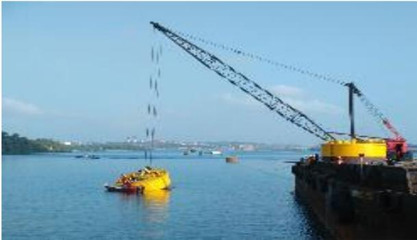
**Gambar 1 .** Proses loading SBM
